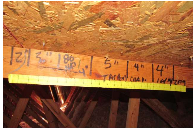
Roof Deck Connection - Nail Spacing #2
