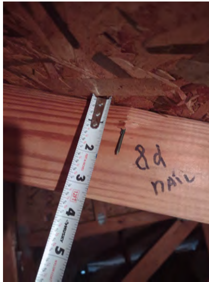
Roof Deck Connection 8D Nail
