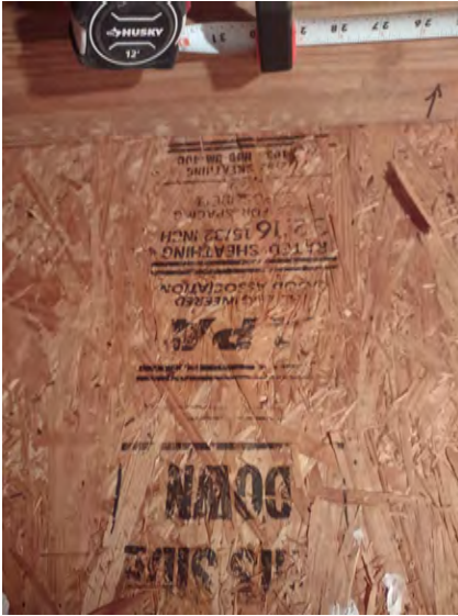
Roof Deck Thickness
