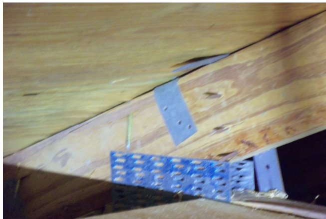
Roof To Wall Attachment - Clips - Back
