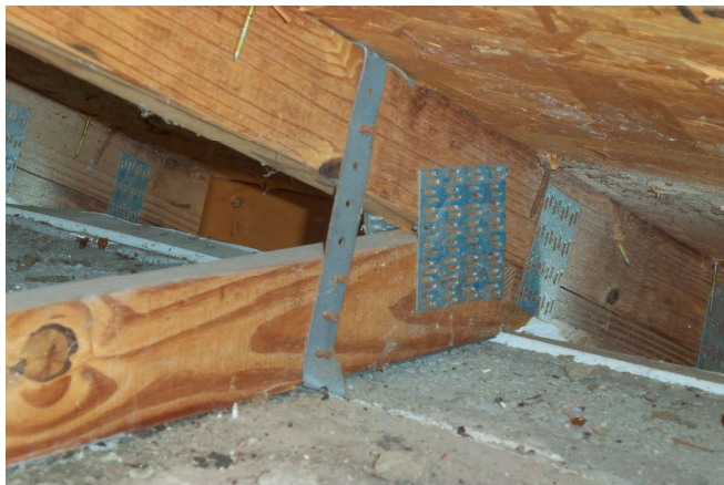
Roof To Wall Attachment - Clips - Front
