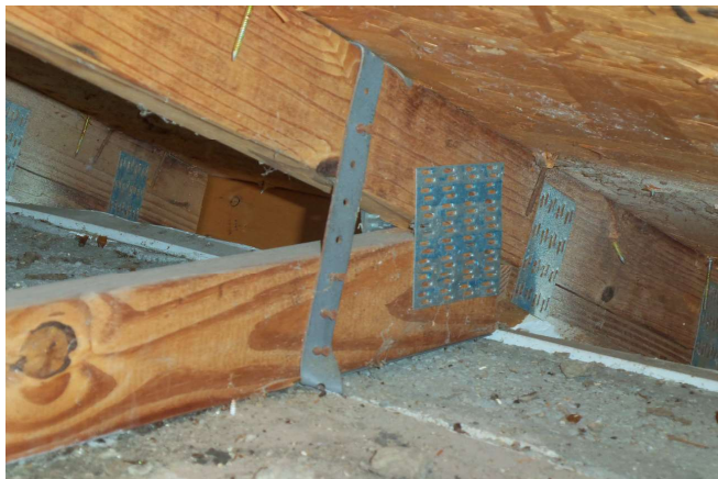
Roof To Wall Attachment - Clips - Front
