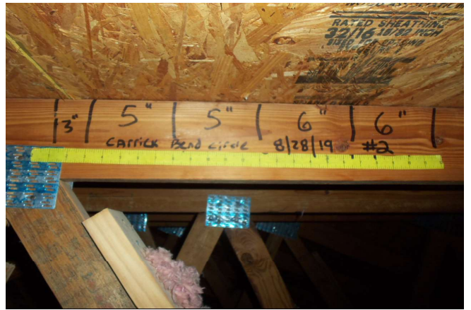
Roof Deck Attachment - Nail Spacing #2
