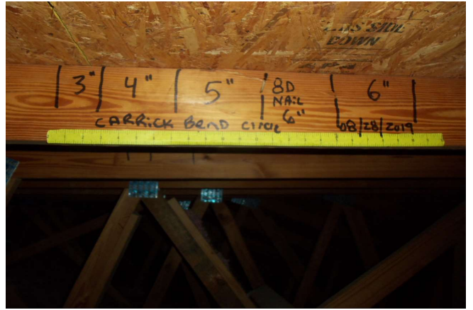
Roof Deck Attachment - Nail Spacing #1
