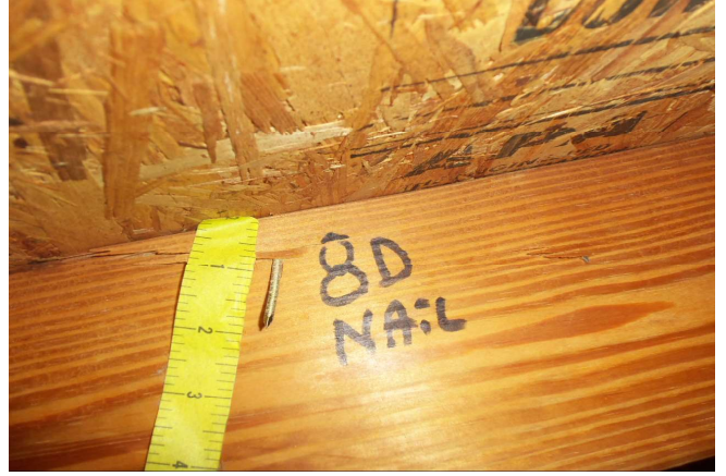
Roof Deck Attachment - 8D Nail
