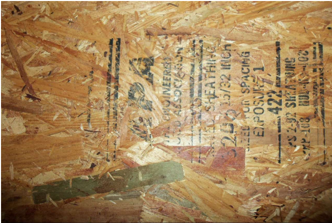
Roof Deck Thickness - 15/32"
