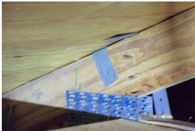
Roof To Wall Attachment - Clips - Back
