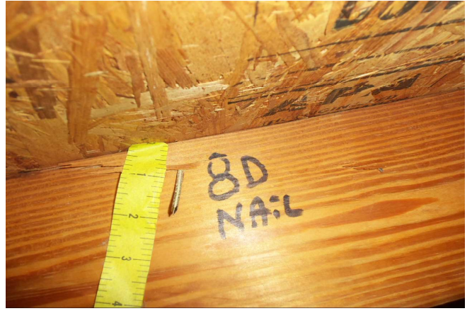
Roof Deck Attachment - 8D Nail
