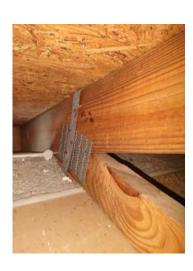
Roof to Wall Connection Single Wrap Front
