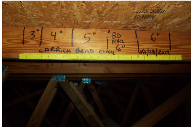
Roof Deck Attachment - Nail Spacing #1
