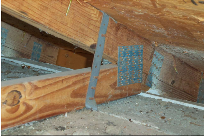
Roof To Wall Attachment - Clips - Front
