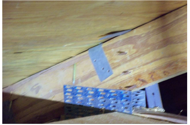
Roof To Wall Attachment - Clips - Back
