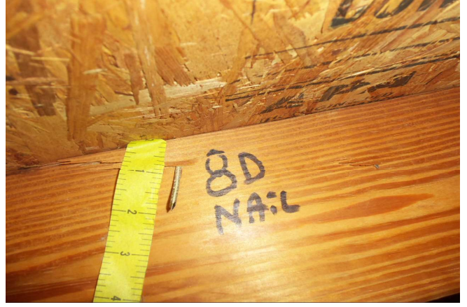
Roof Deck Attachment - 8D Nail
