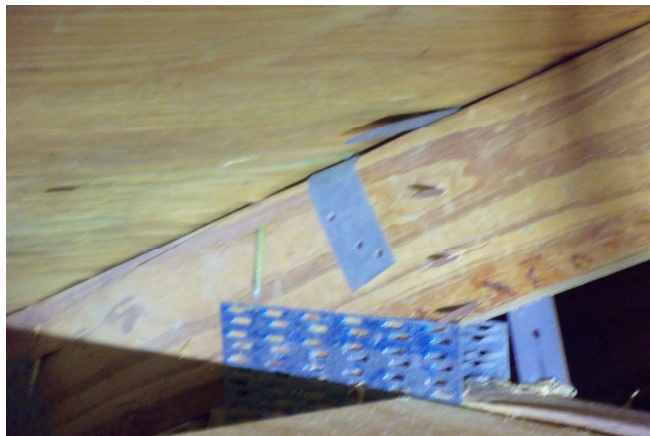
Roof To Wall Attachment - Clips - Back
