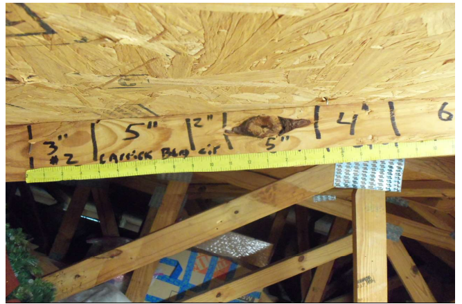
Roof Deck Attachment - Nail Spacing #2
