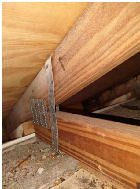
Roof to Wall Connection Single Wrap Front
