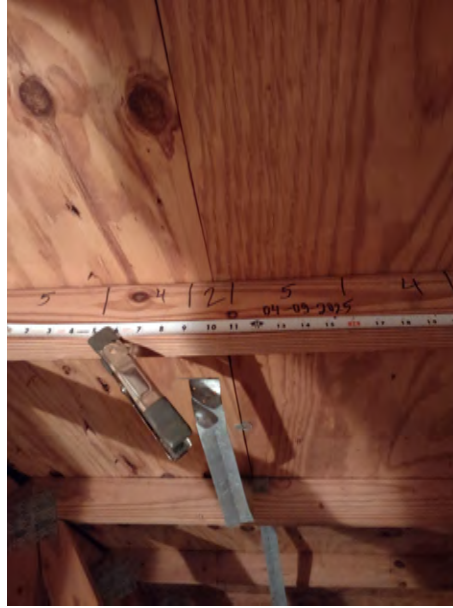
Roof Deck Connection Nail Spacing
