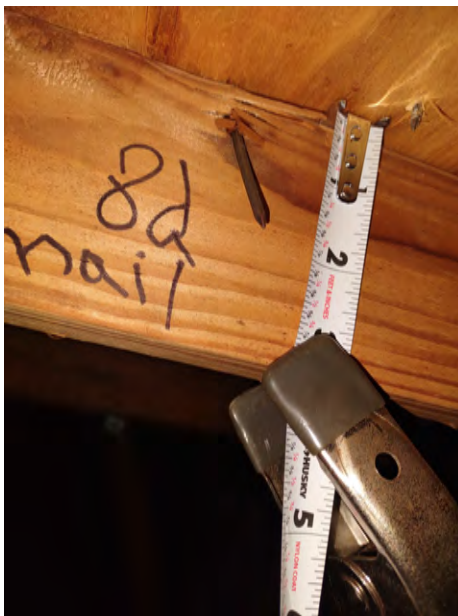
Roof Deck Connection 8D Nail
