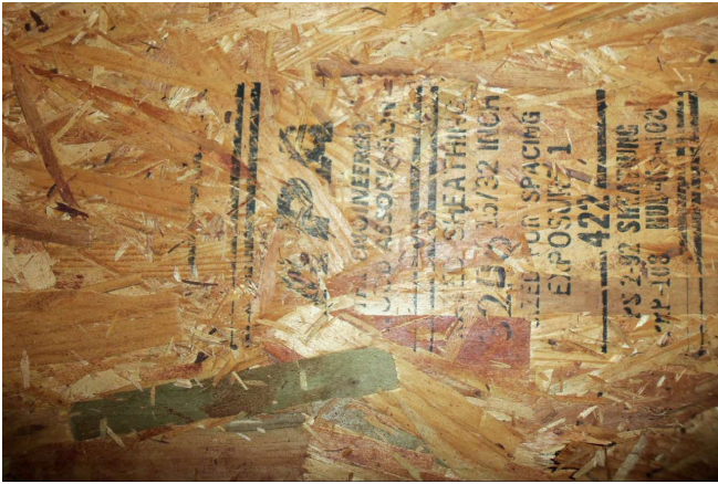
Roof Deck Thickness - 15/32"
