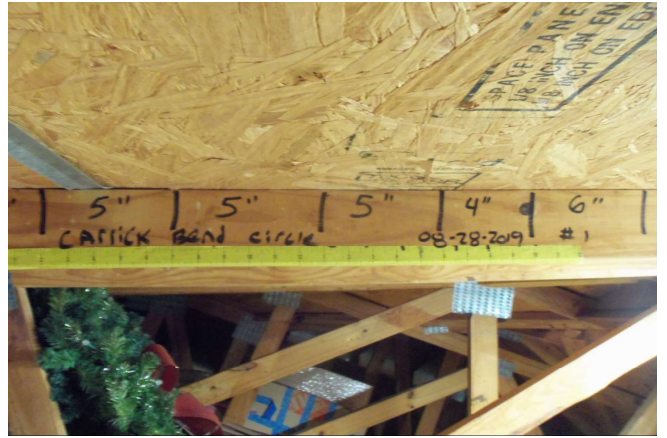
Roof Deck Attachment - Nail Spacing #1
