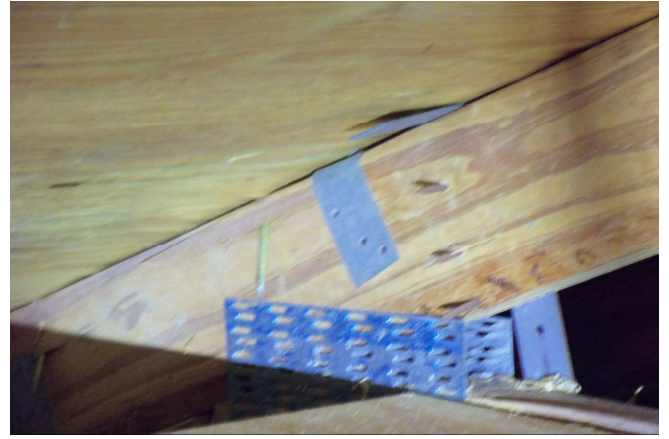
Roof To Wall Attachment - Clips - Back
