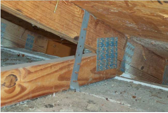
Roof To Wall Attachment - Clips - Front
