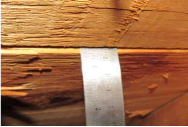
Roof deck thickness - 1/2"
