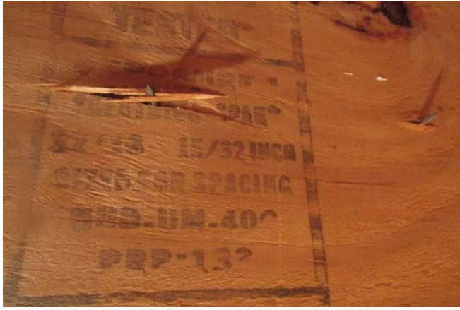
Roof deck thickness - 15/32"
