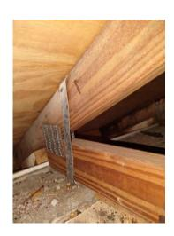
Roof to Wall Connection Single Wrap Front
